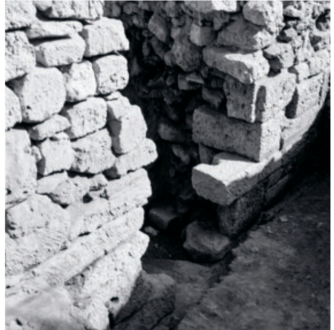
Fig. 17. City wall II façade, excavation through wall at section 3, looking SE. To the right, ashlar with round cutting and rabbet (1961/62).
