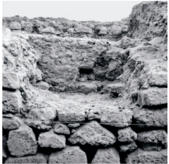
Fig. 10. Early stage of excavation through the city wall at section 3, looking E. In foreground, ashlar façade of wall II. In centre, plastered façade of wall I. In background, above, heavy wall of large stones (1961/62).
