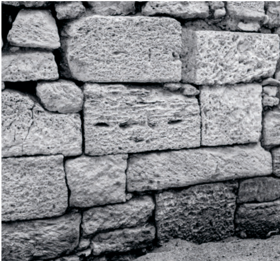
Fig. 13. Ashlars in façade of city wall II, looking E, cf. elevation 1 (1960).
