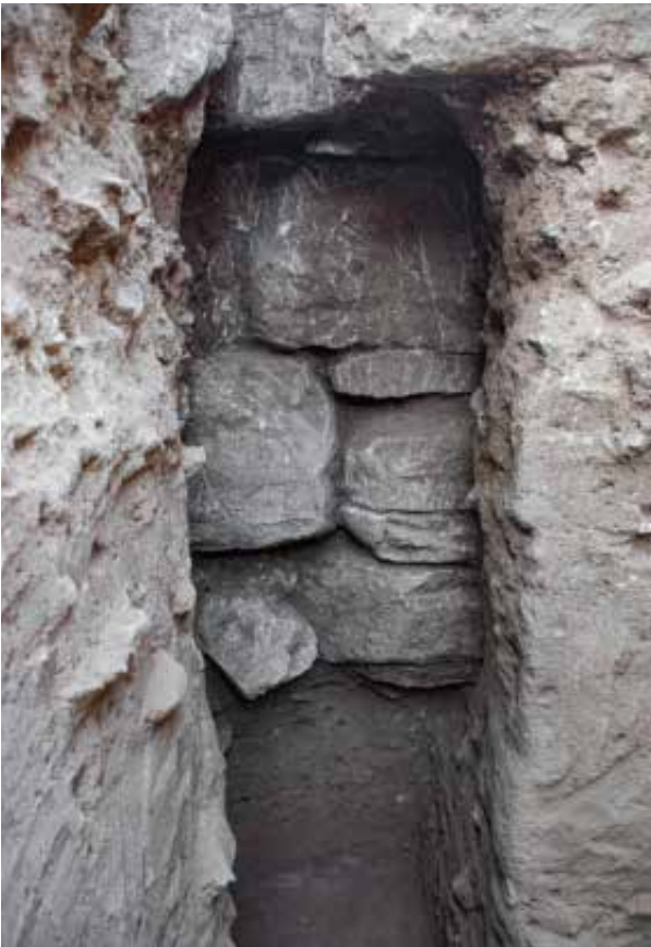
Fig. 2.c.2 Lowest courses of Skene South Wall. From the north, inside the skene, at Z29S (NS section).
