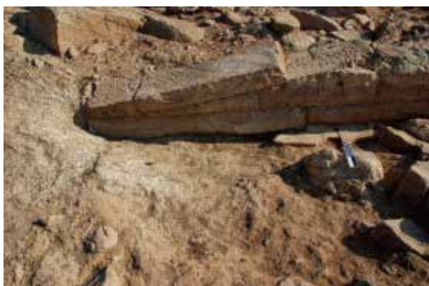
Fig. 2c.21 West end of West Ramp South Wall from the south. Masonry with cover blocks.
