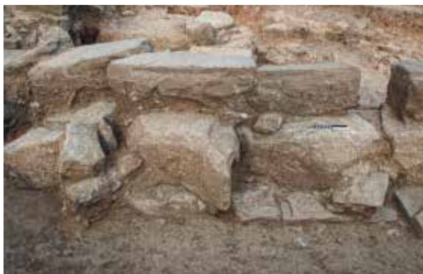
Fig. 2.b.6 Trench A41W with Orchestra Terrace Wall seen from the west. Drafting to mark the level of the orchestra level at upper edge of blocks is visible.
