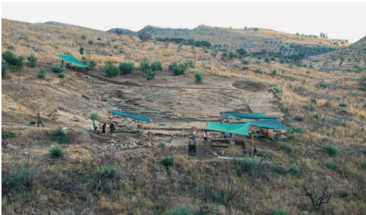
Fig. 1.5 Excavation in progress, July 2012. It is clearly visible how the exposed layers of bed rock are responsible for the shape of the hill side and how they continue sloping downwards in eastern direction beyond the excavation.
