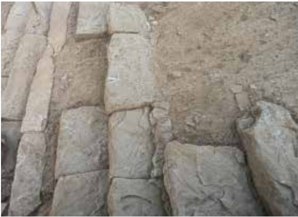
Fig. 2.a.6 Detail of koilon. Nature of preservation and weathering of seats blocks in lower east half of central area. Flaking obvious on blocks IV.27 and 28. From the east.
