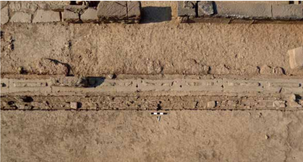
Fig. 2.c.15 Central part of proskenion stylobate, south is up. Rhombus-shaped dowel holes, curbs and circular cavities visible. South is up.
