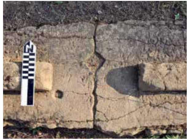
Fig. 2.c.14 Detail of proskenion stylobate showing the structure and colour of the sandstone and surface treatment as preparation for installation of pilaster.
