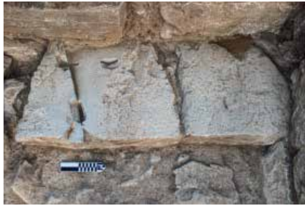
Fig. 2.b.4 AS31 seen from the east. Above the lowest part of the Orchestra Terrace Wall is visible.
